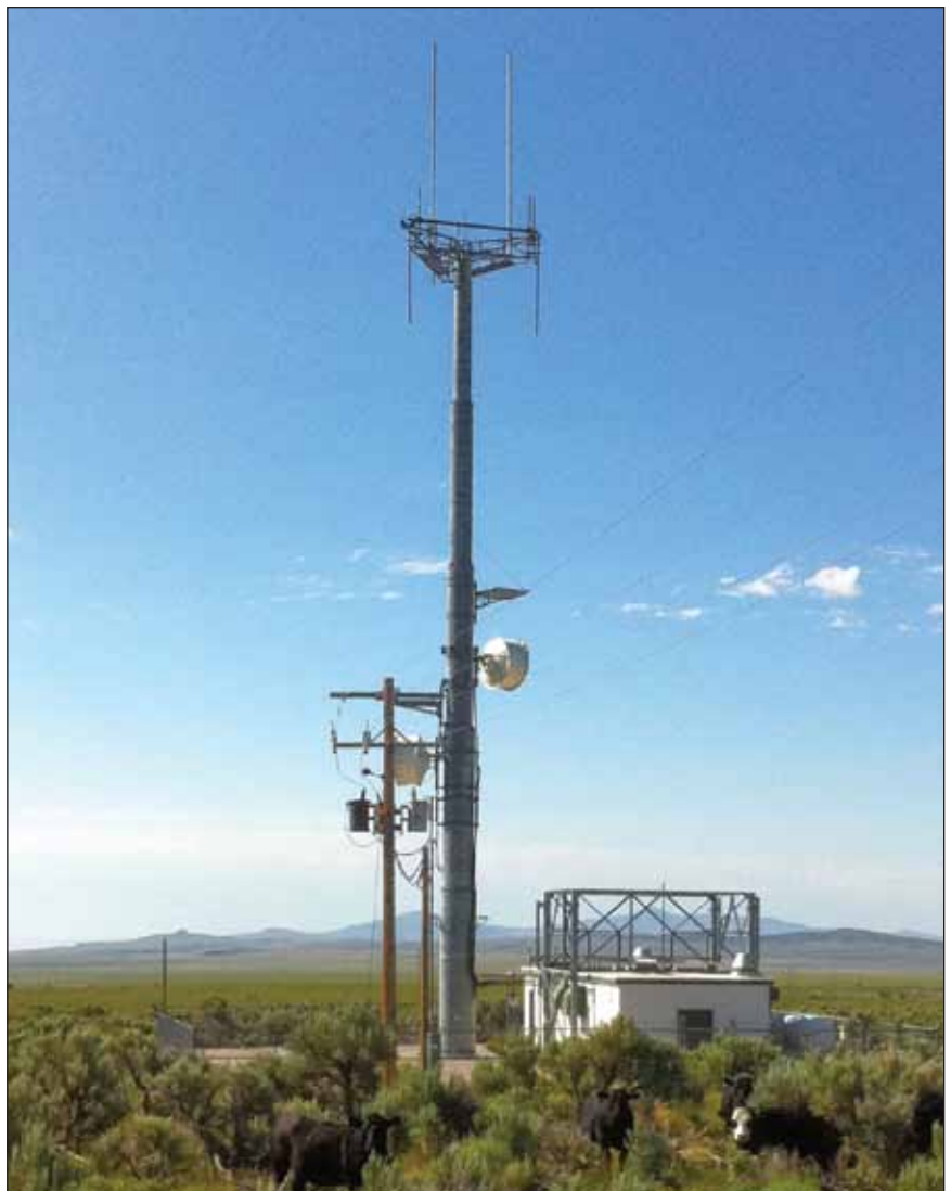
Cell tower in northwestern Utah near Park Valley, pop. 270 (nowhere near Park City) with curious cattle looking on.
